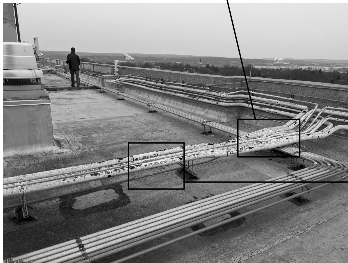
E REFRIGERANT MAINS AND REFNET FITTINGS, SYSTEM #4
